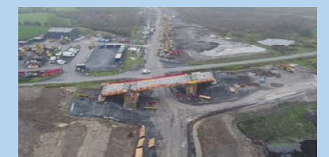
Structure 7—Drumfin Overbridge (South)
