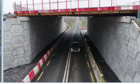
Structure 11—Ardloy Underbridge
