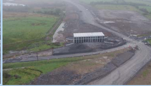
Structure 10—Kingsbrook Underbridge
