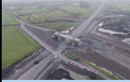
Structure 6—Drumfin Overbridge (North)
