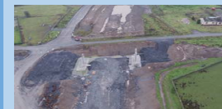
Structure 4—Knocknagroagh Overbridge
